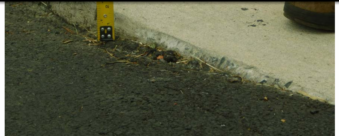
Figure 3.1.5.2.2 Beveled Change in Level (R302.7.2)
