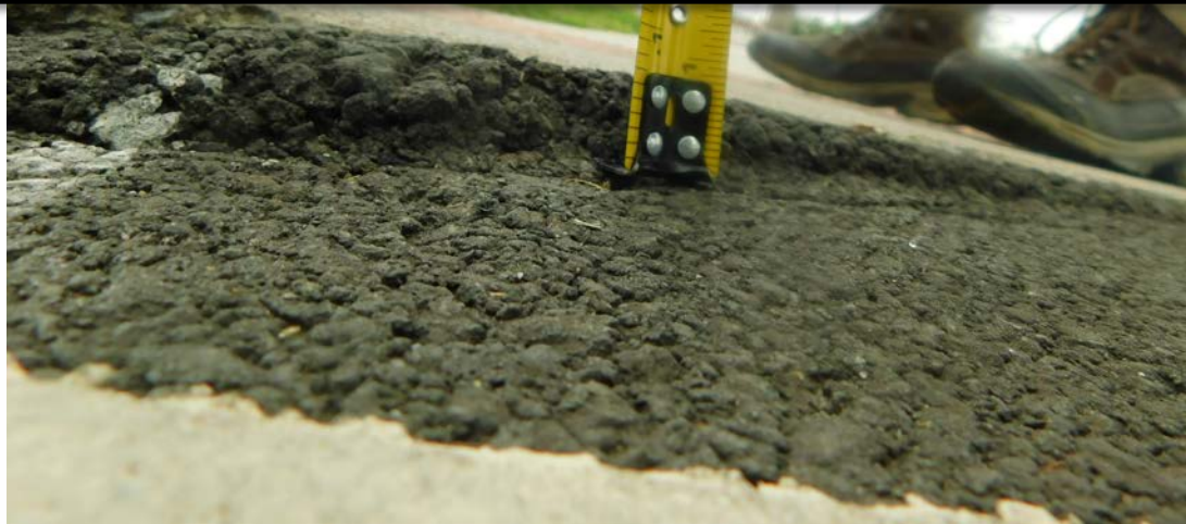
Figure 3.1.5.2.1 Vertical Change in Level (303.2)
